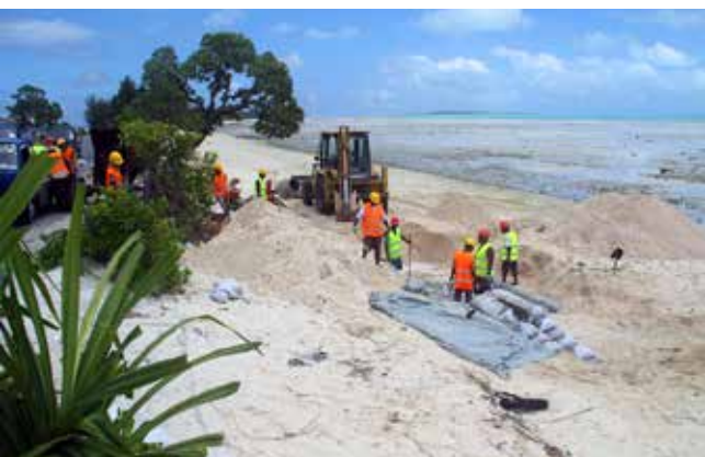
Seawall installation in Bairiki Nanikaai Causeway, Kiribati (GEF)
