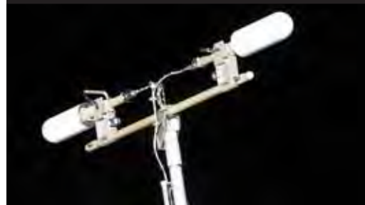
UHF antenna on the P1 Truss.
